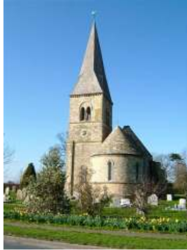
August 2005 - Work to Apse roof is undertaken
