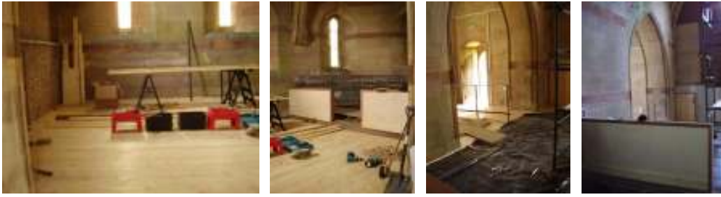
Internal Views of Chancel and vestry May 2006
